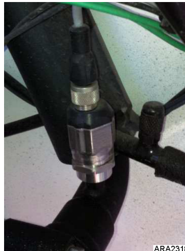
Suction Transducer Installed
