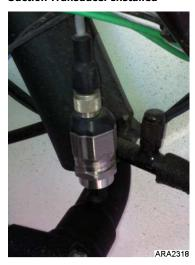
The Low Pressure Cutout Switch or Suction Transducer will have the same function, since the unit only has one fitting on the suction tube, the unit can have either a Low Pressure Cutout Switch or Suction Transducer but not both.
