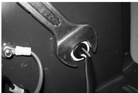
Figure 6: Tighten Bulkhead
